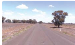
Newell Highway north of Finley — No delineation, unsealed shoulder, undivided, good roadside condition and good horizontal alignment
