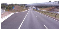
WestLink M7 — Good horizontal alignment, good delineation, divided, overpass intersections and excellent overtaking opportunities
