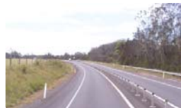
Pacific Highway south of Nambucca Heads — Innovative use of wire rope barrier to create a divided road, good delineation, moderate roadside severity, gradual bend
