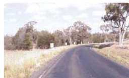
Mitchell Highway west of Orange — Poor delineation, poor horizontal alignment, undivided, no overtaking opportunity
