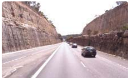
F3 south of the Hawkesbury River — Severe roadside conditions, good alignment, divided, excellent overtaking opportunities, mountainous terrain
