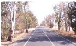
Barton Highway near Murrumbateman — Severe roadside condition, undivided, good delineation and good horizontal alignment
