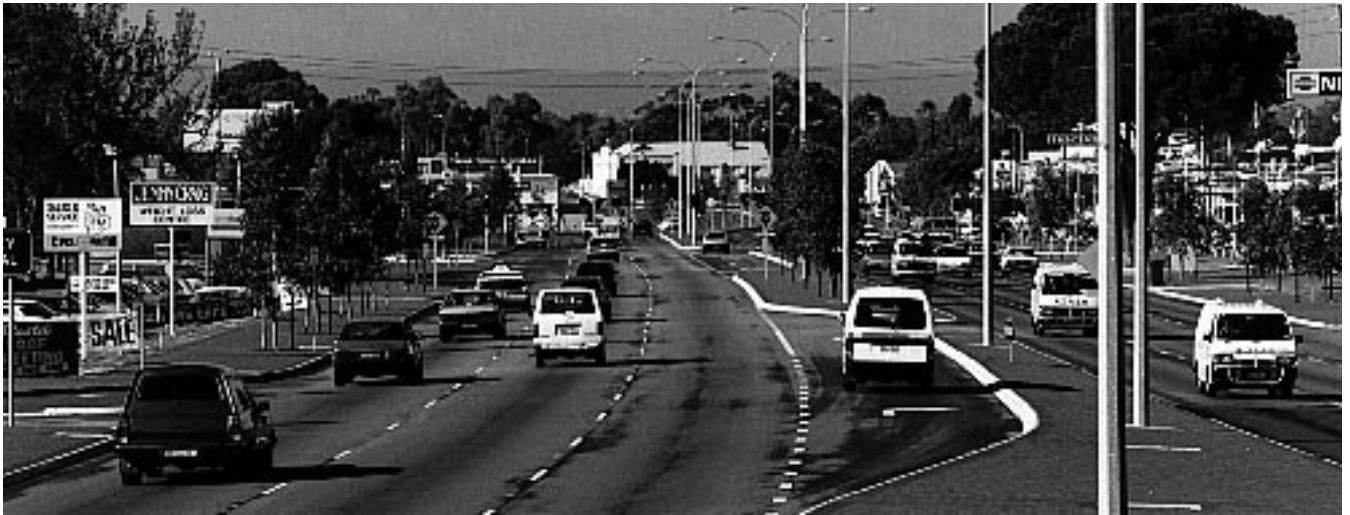
A section of the Albany Highway at Cannington, WA, recently widened and improved under the state's 10-year road program.
